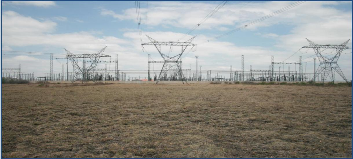
**Figure 3:** Bighorn –Marang and Medupi-Marang 400kV power lines feeding into Marang MTS
